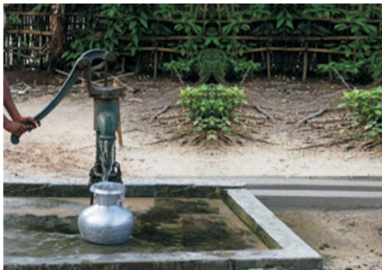
Fig. 1.3: Proper drainage of water near the hand pump, taps and wells
