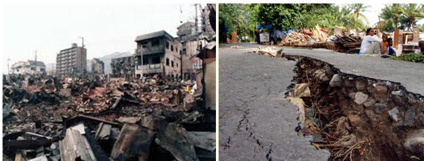
Fig. 30.3 Collapsing of buildings and build up debris
