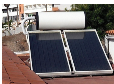
Fig. 12.3 Solar flat plate collector
